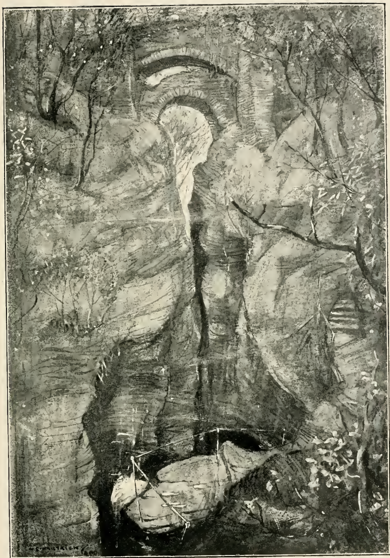
THE DEVIL'S BRIDGE.
